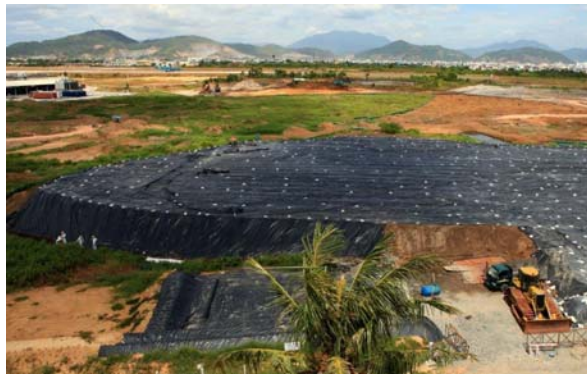
Temporary storage of Phase 2 material (Photo: Tetra Tech)
