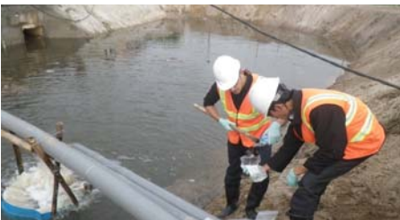
Sampling water to ensure contamination does not leave Project site (Photo: CDM Smith)
