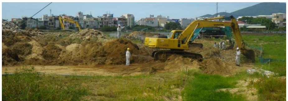
Excavating Phase 2 soil and sediment
