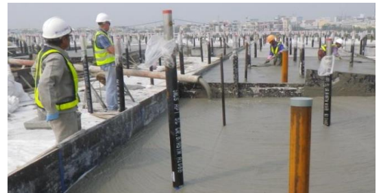
Pouring concrete cap on top of containment structure (Photo: CDM Smith)
