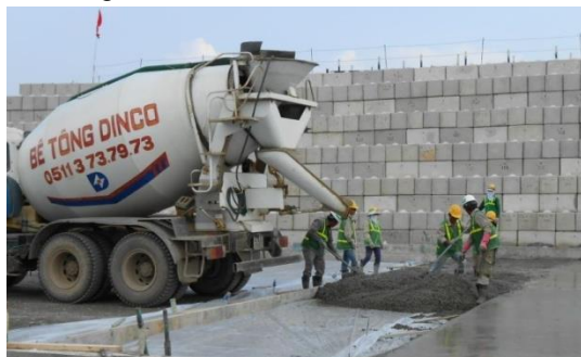
Building foundation of liquid and vapor treatment system (Photo: CDM Smith)
