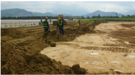
Backfilling at the former Mixing and Loading Area (Photo: CDM Smith)
