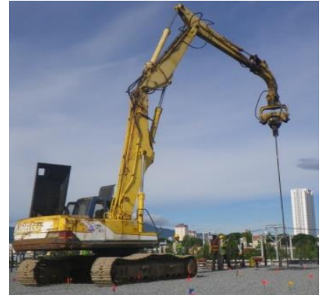
Installing heater cans into the containment structure
